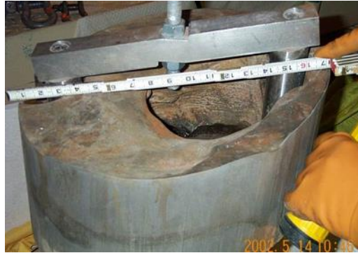
Figure V-1: Davis Besse RPV Head corrosion effects
